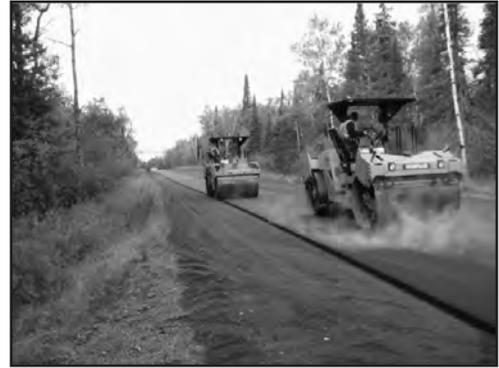
**Solution** Lake County developed potential reclaimed asphalt pavement (RAP) mixes containing imported, high-quality aggregates that could be tested in a low-volume pavement project. These mixes allowed the county to reduce the amount of new asphalt needed while also using surplus RAP material available from local surface renewal projects. The addition of high-quality aggregates also provided a more durable bituminous surface.
