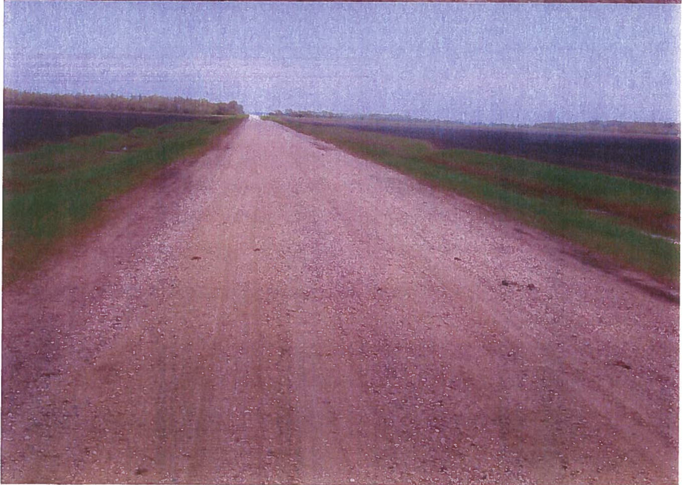
Road Preparation before adding MgCl_2
