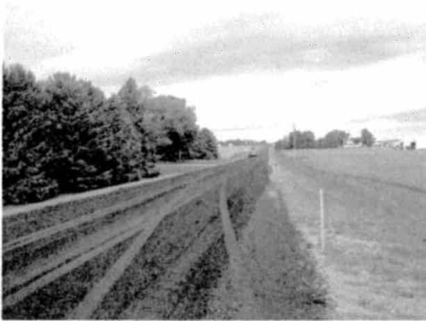
Placing RAS/RAP Blend with Blade
