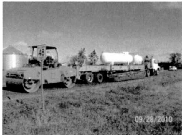
Heating and Compacting Surface
