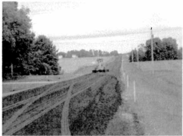
Placing RAS/RAP Blend with Blade
