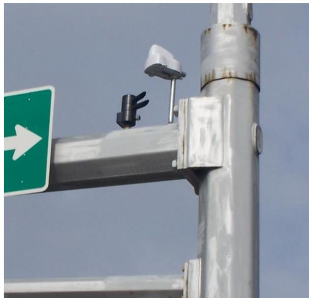
**Figure 4: GPS and optical preemption devices on traffic signal arm**
