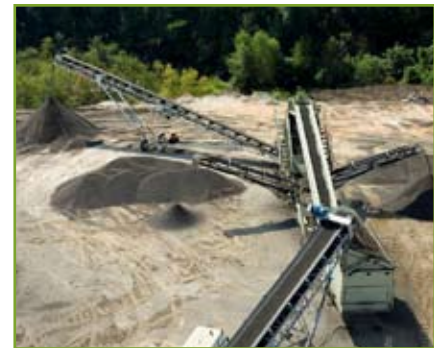
RAP segregated in piles
