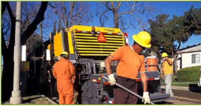
Rubberized slurry seal in Los Angeles
