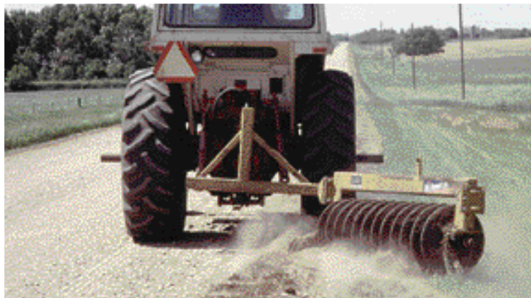
Same machine mounted on a farm tractor to help break up material on shoulder.
