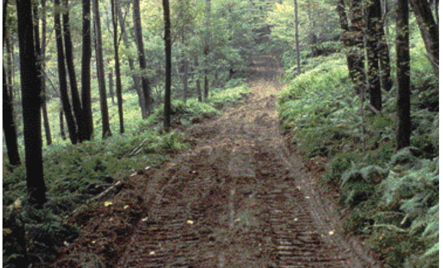
This gravel road with narrow right-of-way has turned to mud during wet spring conditions. It represents low-volume roads commonly found in several parts of the world.
