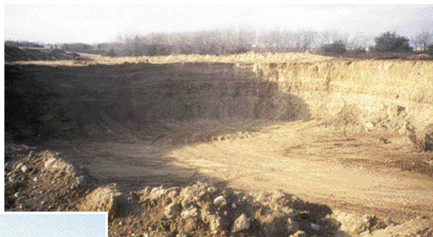
A good example of topsoil and vegetation that has been stripped from the surface of a gravel pit and placed beyond the working area. It can later be placed back over the bottom of the pit as part of the reclamation process. It will once again grow grass.
