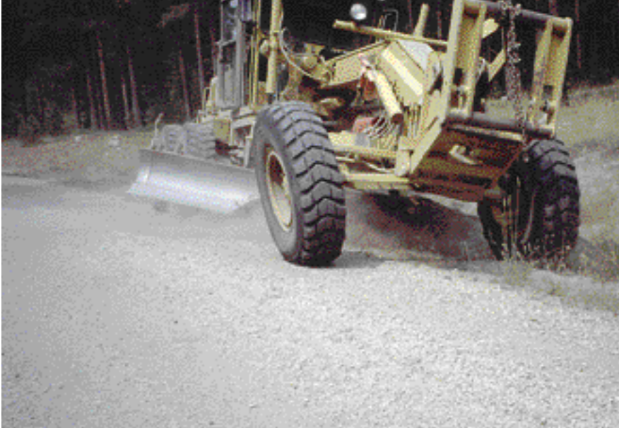
An example of work with a grader to reshape a ditch on a mountain road.
