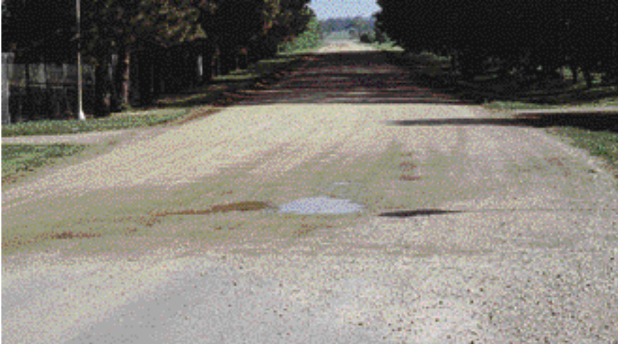
It is a good practice to loosen, mix, reshape gravel in a washboard-prone area while it is moist.
