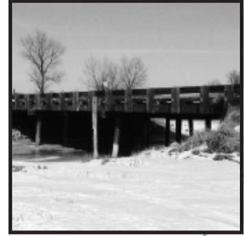
**Problem** Owners of the approximately 1,300 treated timber bridges in Minnesota are looking for inexpensive and easy ways to increase the load capacity and serviceability of existing timber bridges to accommodate both the increased number and size of vehicles now depending on local road systems.
