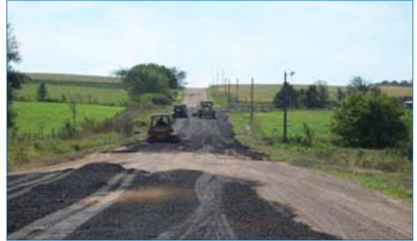
Problem Water that seeps into gravel or red rock roadbeds can cause frost boils and other road defects, as happened on heavily traveled Scott County roads on a yearly basis. These road conditions resulted in complaints and shoulder damage.
