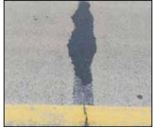
**Problem** Extensive cupping at transverse cracks in bituminous pavements allows water intrusion and accelerates pavement deterioration. It also makes for a rough ride for drivers. A more cost-effective repair strategy is sought in lieu of a traditional mill and overlay to eliminate cracks and improve ride.
