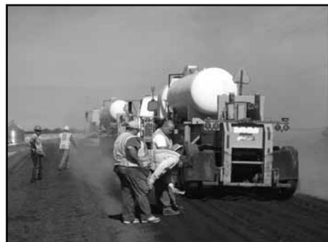
**Solution** Blue Earth County completed a gravel road stabilization project on a section of County State Aid Highway (CSAH) 48 using a blend of recycled asphalt shingles (RAS) and recycled asphalt pavement (RAP) rather than the typical stabilizing binder used in past projects. This mix required almost a third less asphalt emulsion than bituminous stabilized gravel roads.
