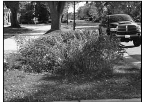
**Problem** Increased environmental awareness has led local roadway agencies to consider various means of mitigating the effects of stormwater discharge into lakes and rivers. One technique is to install rain gardens that partially treat the stormwater. Unfortunately, many urban settings do not have enough space to construct a rain garden large enough to fully absorb storm runoff.
