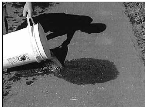
**Problem** Sealing asphalt pavements typically requires the application of petroleum-based products, which can be harmful and inconvenient in areas with high volumes of pedestrian traffic.
