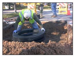
**Problem** The traditional method of adjusting the elevation of a manhole casting by using concrete
